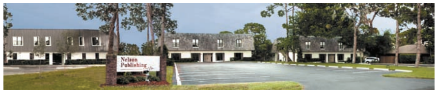
Nelson Publishing, Inc. Headquarters • Nokomis, Florida
